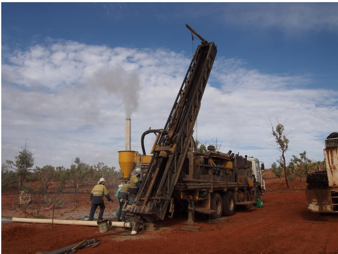
Figure 1. Drilling Commences (RC Rig in operation)
